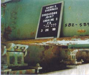
Deteriorated bearings.
